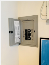
Circuit breaker panel within apartments
